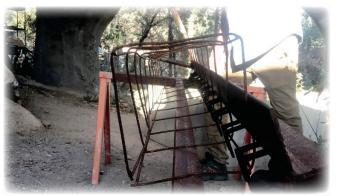
The Precision Contour Control Framing represents about 1/3 to 1/2 of the labor for the finished product. It takes about a week to do the framing for a small Flex-Shell Core Monolith Pavilion home, while the lath fabric and plaster shell take the remaining time.
